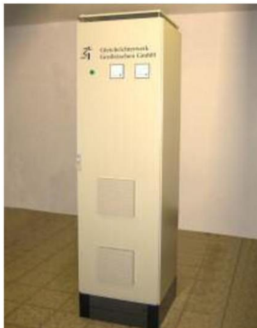
DC-Anlage 40Vdc / 400Adc
